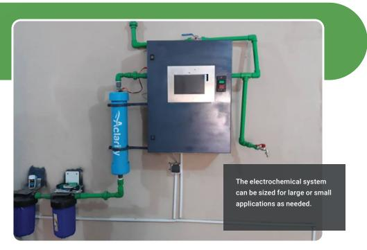
or near the electrode surface. At low voltages, around 6 volts, oxidants, such as hypochlorite and hydrogen peroxide are generated.
